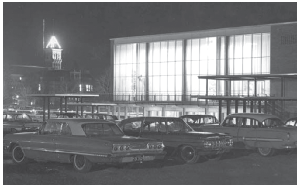
In recent decades, the building now known as the Taggart Student Center has become home to various administrative offices and student-facing departments, while still playing a pivotal role for student activities. Photos courtesy of USU Merrill-Cazier Library, Special Collections & Archives.
