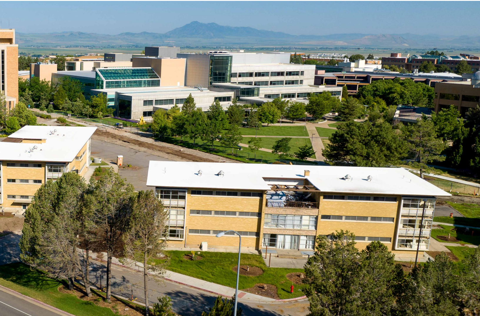
Initially built in 1955 as women-only dormitories, the Reeder, Greaves, and Moen residence halls are being torn down to make way for three new campus structures. Those include a new five-story housing facility, a parking structure, and the Kem and Carolyn Gardner Learning and Leadership Building that will house the Jon M. Huntsman School of Business’ experiential learning program. Photo by Levi Sim.
